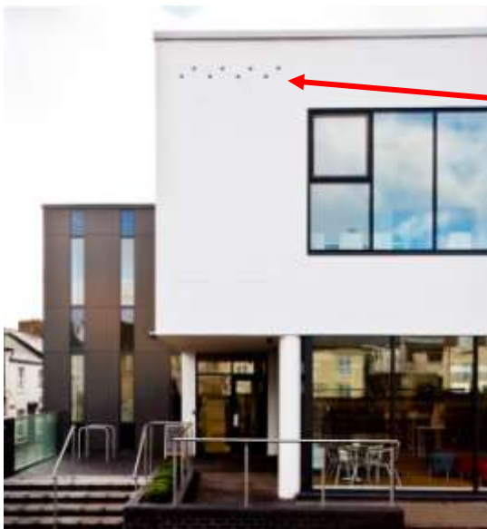
Eight Schwegler Swift Bricks were installed and hidden behind the plastered facade of the new Cullompton Library in Devon
