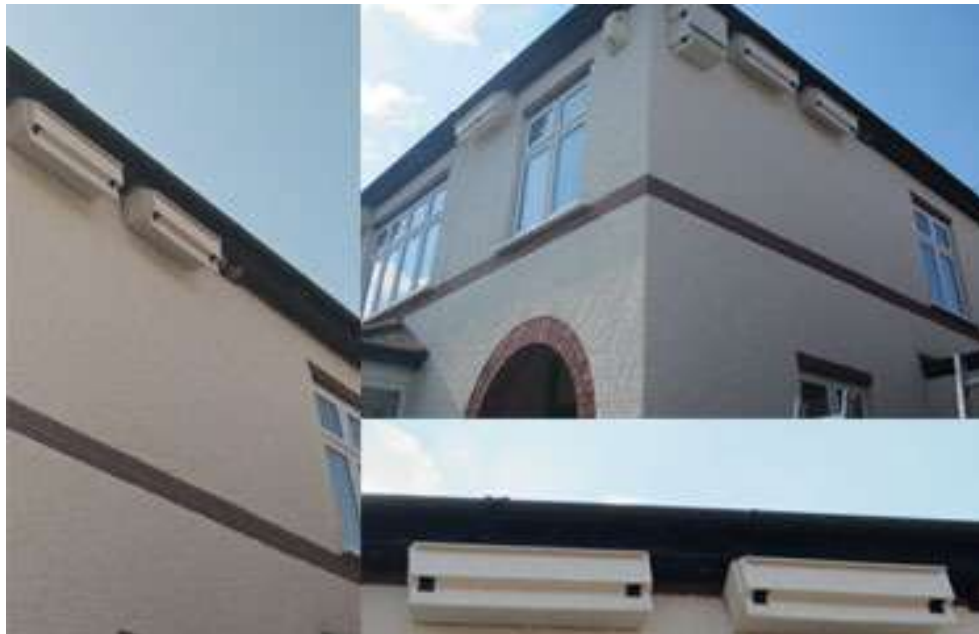
Photos showing finished boxes in position
