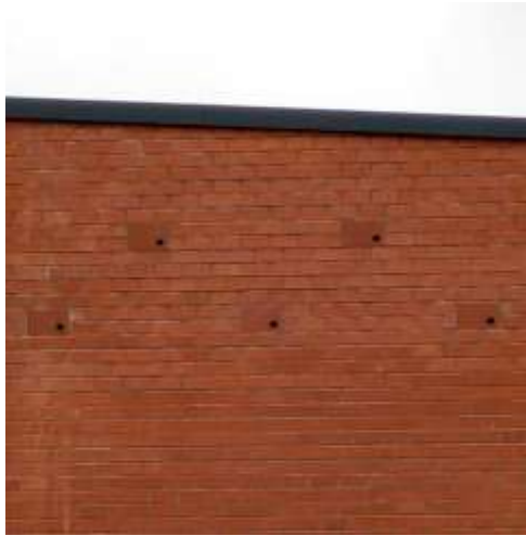
Antrim Public Library, Northern Ireland: Istock Swift bricks were used to bring life to this featureless wall
