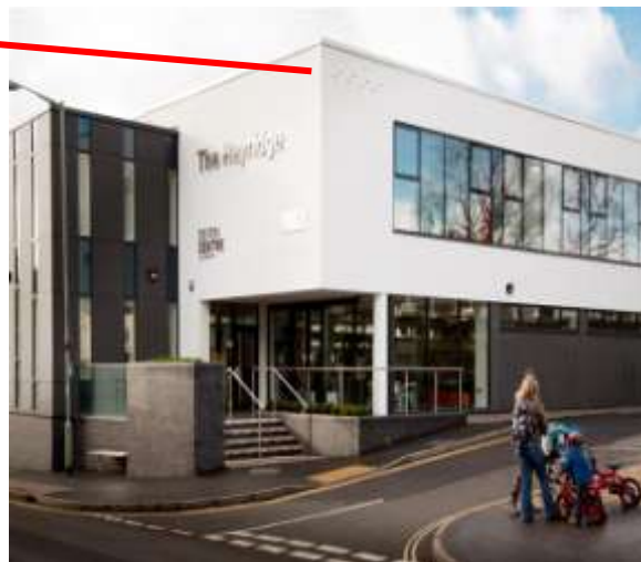
The New Library at Cullompton - the Swift Bricks are scarcely visible but should bring some aerial life and action to this new site
