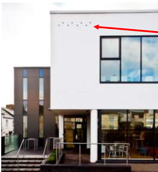
Eight Schwegler Swift Bricks were installed and hidden behind the plastered facade of the new Cullompton Library in Devon
