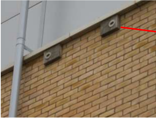
Two Schwegler Swift Bricks installed in the walls of the Maternity Unit at the Lister Hospital
