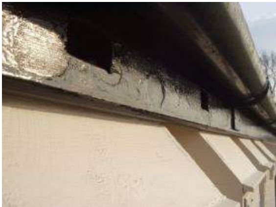
Holes cut in the facing boards let the Swifts reach their nests in the eaves of this chapel Photo © Mark Glanville
