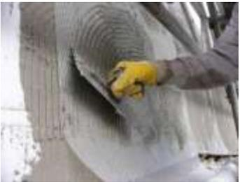
3. Plastering the “Bricks” leaving only the entrance hole visible (see photo on left).
