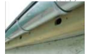
Tailor-made self-contained nesting sites can be created in pitched roofs. In addition openings in the existing fascia boards can be made on the facade.
