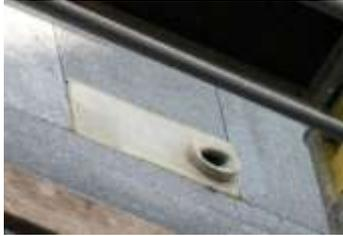
1. Swift “Brick” fitted flush into an exterior facade (see photo on left).
